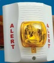
Amber strobe units triggered by the mass notification system accompany the voice instructions to alert occupants that an emergency exists.
